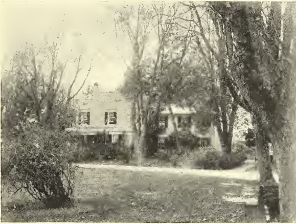
320. THE PRINCIPAL'S HOUSE, HAMPTON An old colonial mansion, dating back to the eighteenth century
