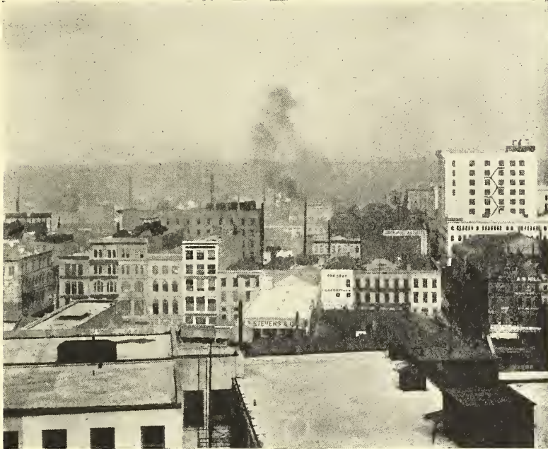
380. NEW ORLEANS FROM AN HOTEL ROOF
