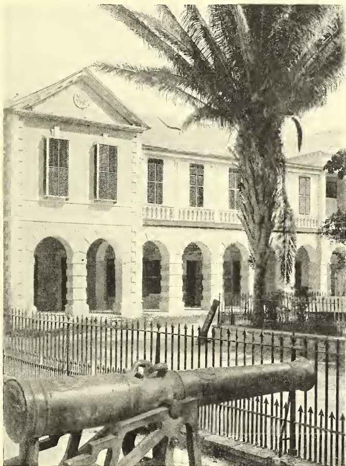
224. THE GOVERNMENT BUILDINGS IN SPANISH TOWN
