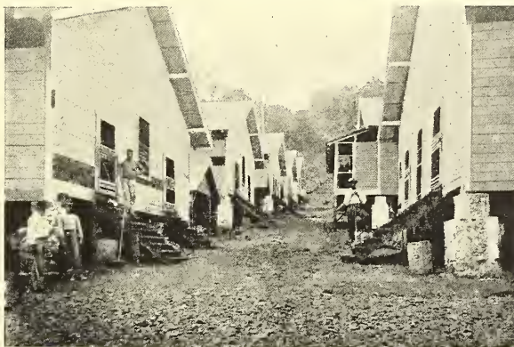
43. NEGRO QUARTERS AT RIO GRANDE, PANAMA CANAL
