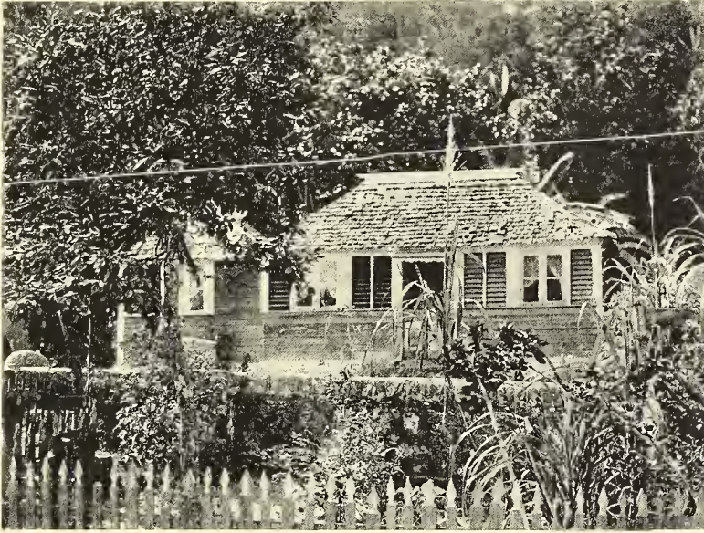
234. THE HOME OF A PROSPEROUS NEGRO PLANTER, JAMAICA Note the telephone wire running past the house, ugly but practical
