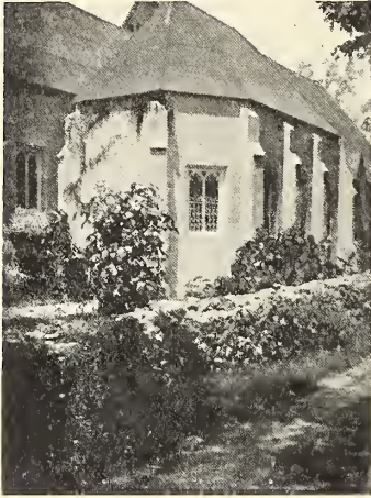
262. A CORNER OF THE EXTERIOR OF THE "COLOURED" PEOPLE'S CHURCH OF ST. AGNES, NASSAU
